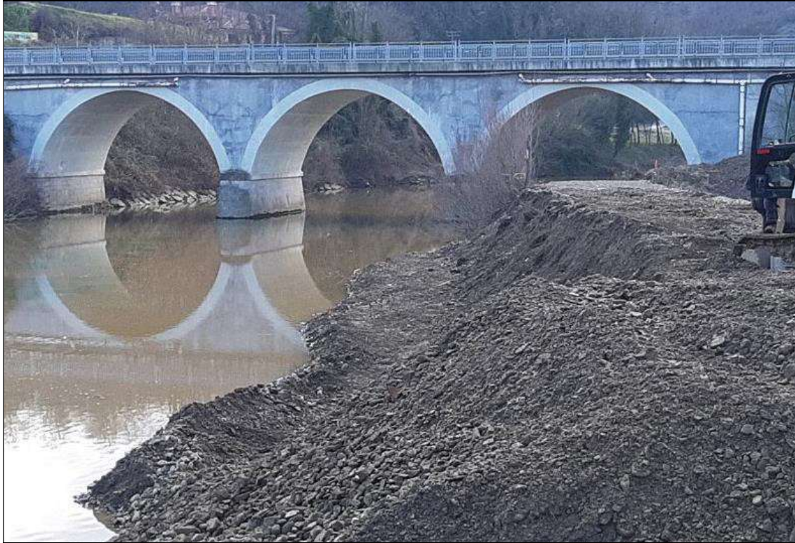
Fig. 7 Construction works for increasing the flood protection of the Draga settlement
