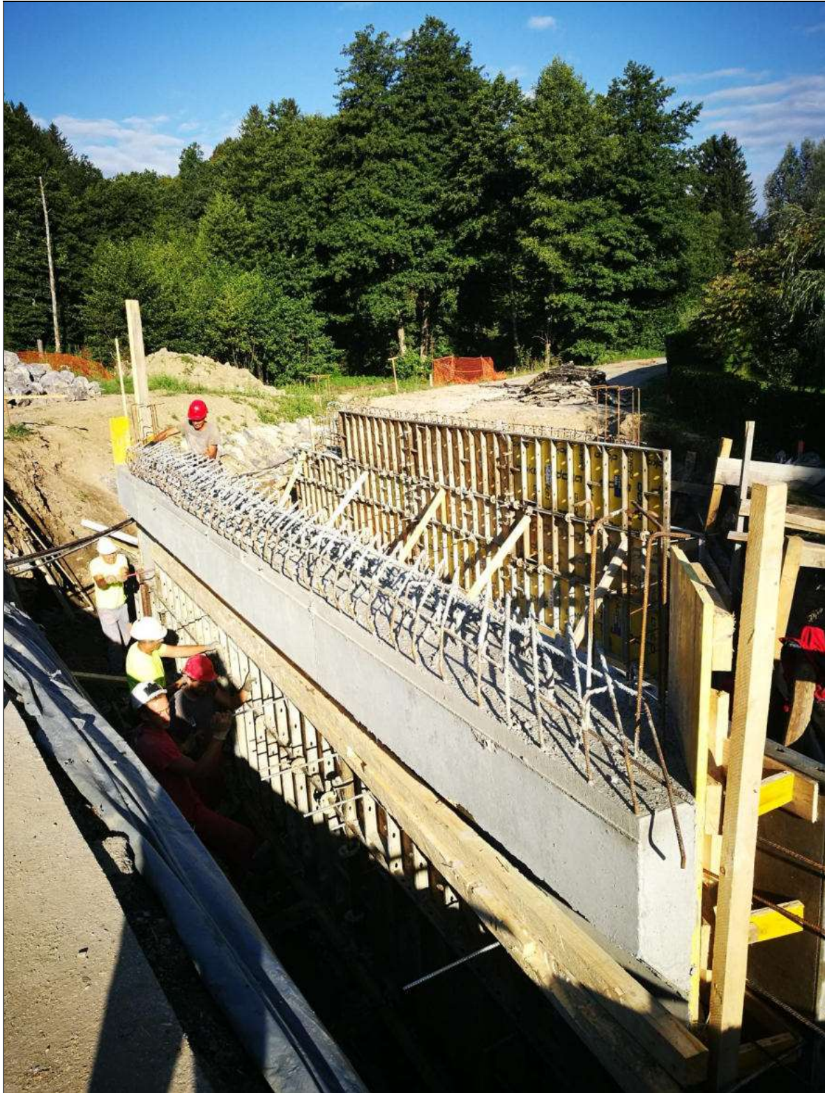
Picture 9: Construction of culvert n. 1
