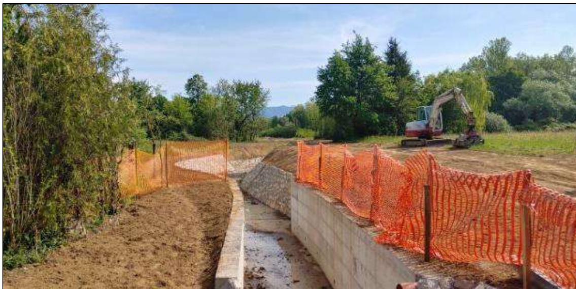
Fig. 10 U-shaped concrete channel construction
