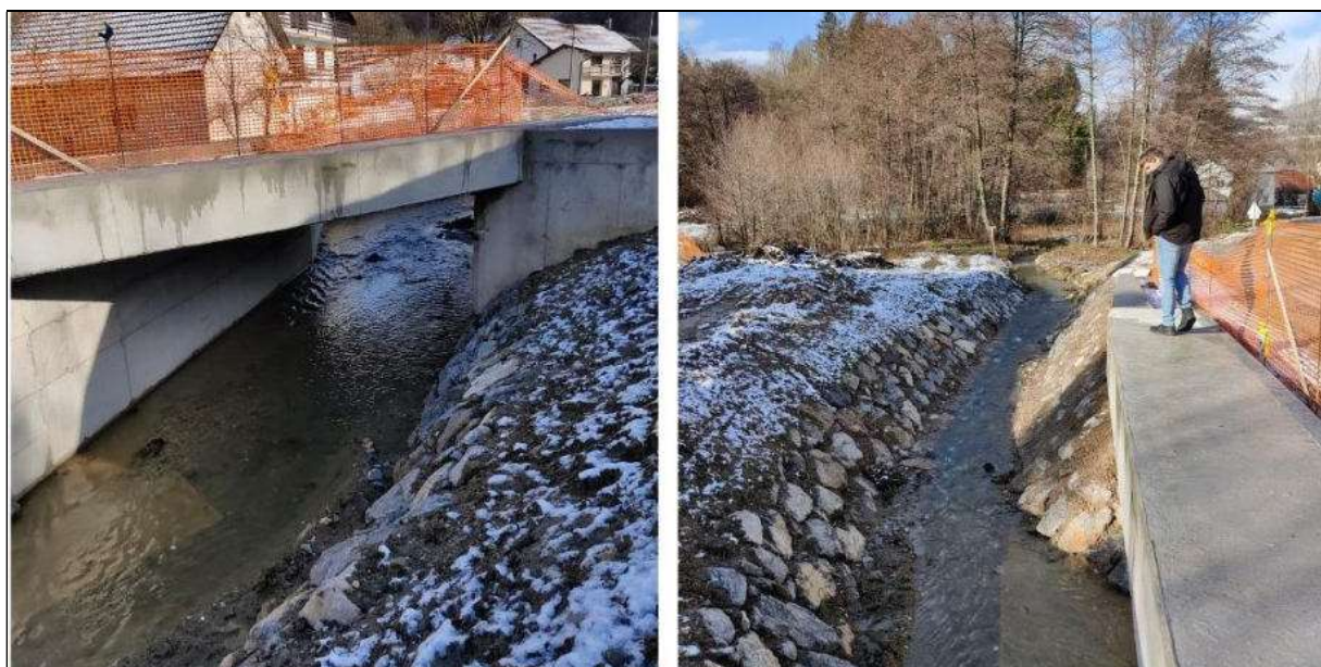
Picture 11: Work before final conclusion
