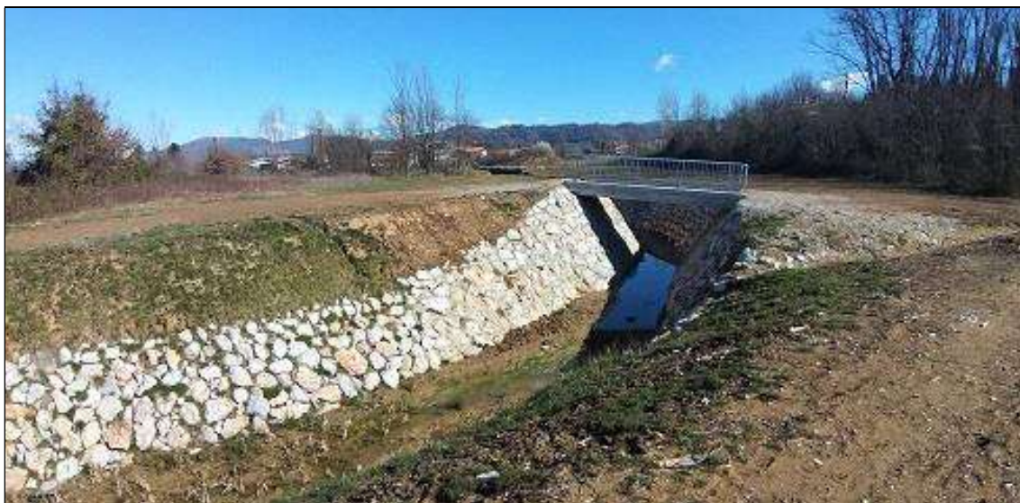
Fig. 11 Adjustment of the culvert into a reinforced concrete bridge
