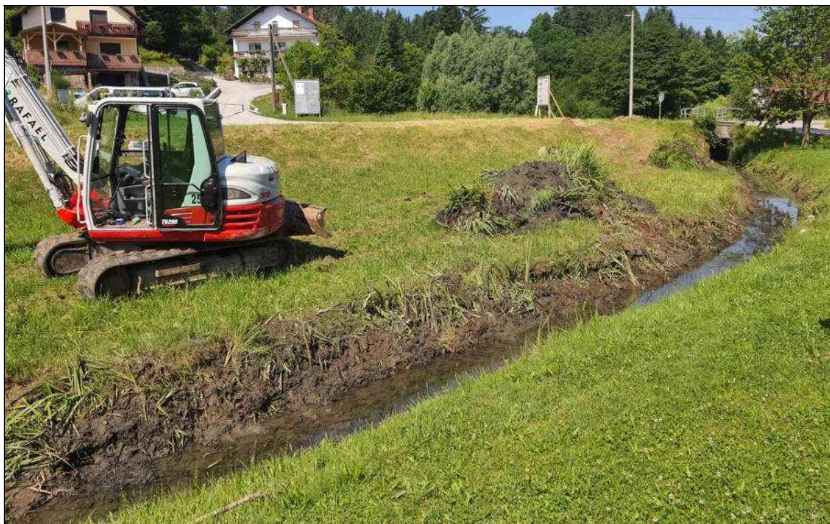
Picture 10: Riverbed before construction
