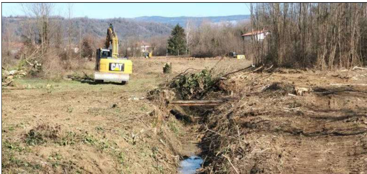
Fig. 8 Construction works: preparation and cleaning of the terrain
