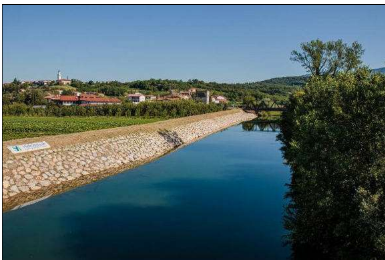
Fig. 9 Finished construction works
