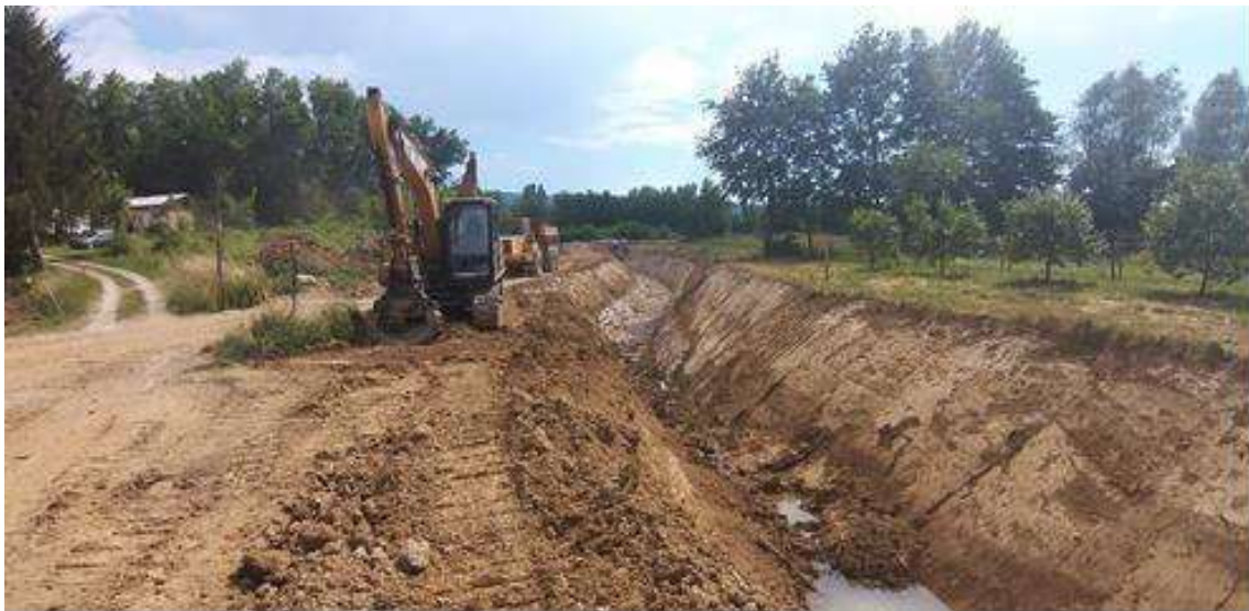
Fig. 9 Enlargement of the section of the watercourse "J2"
