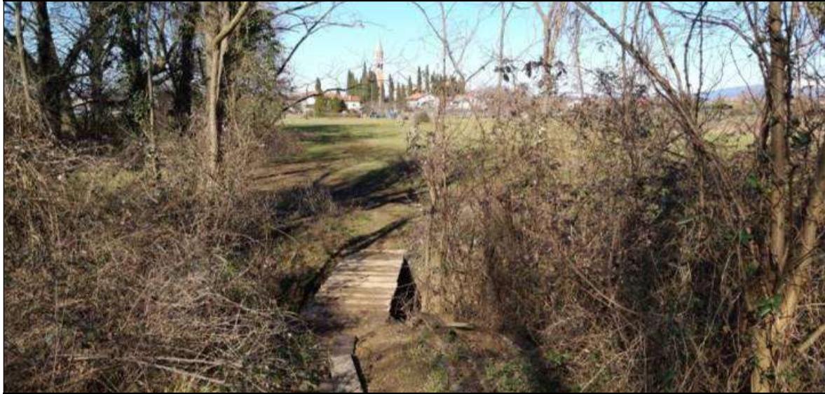
Fig. 7 View of the construction site before starting the works
