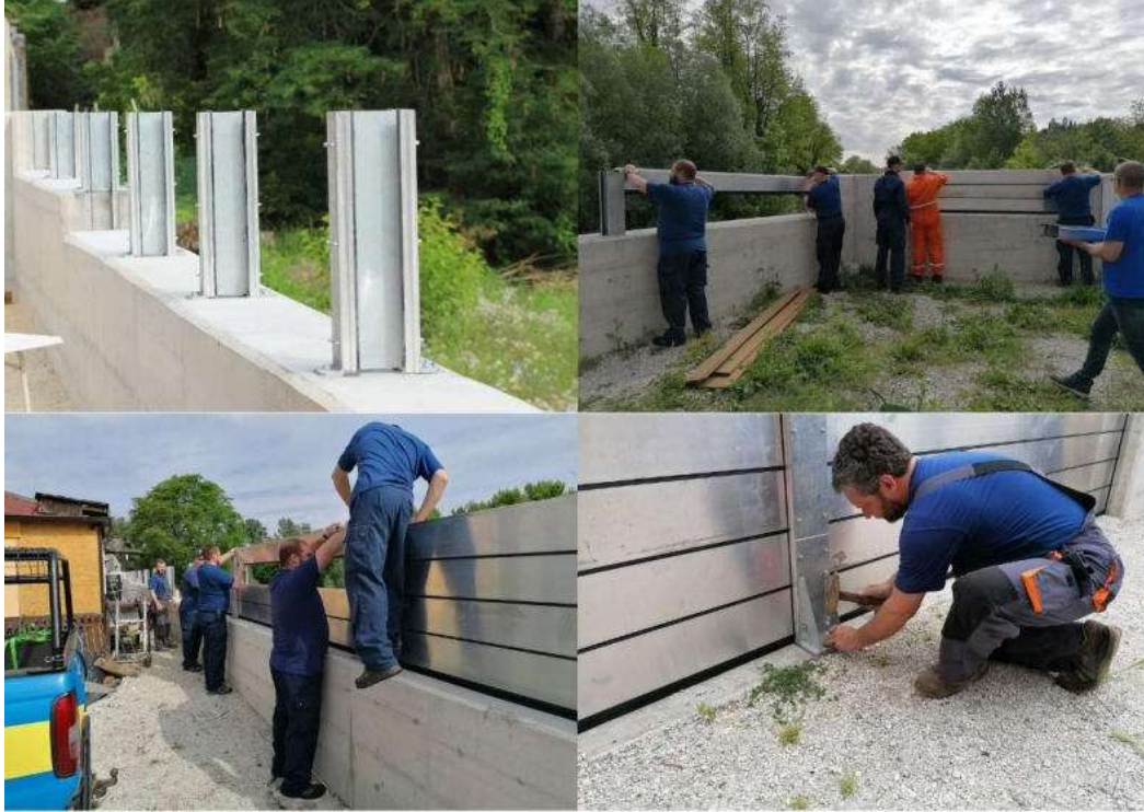
Fig. 12 Mobile gate assembly
