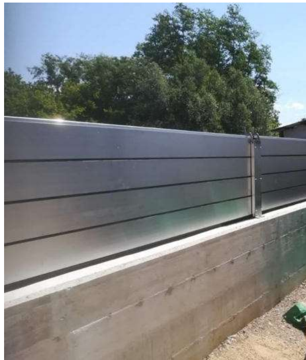
Fig. 13 Mobile gate completed
