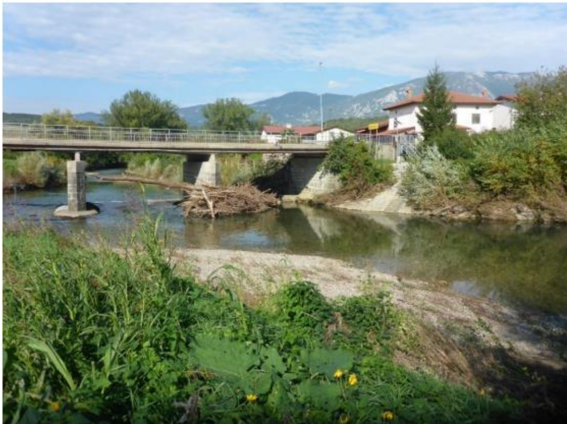
Image 9: Left bank gravel dune in Zalošče upstream of the bridge - proposed exit point.
