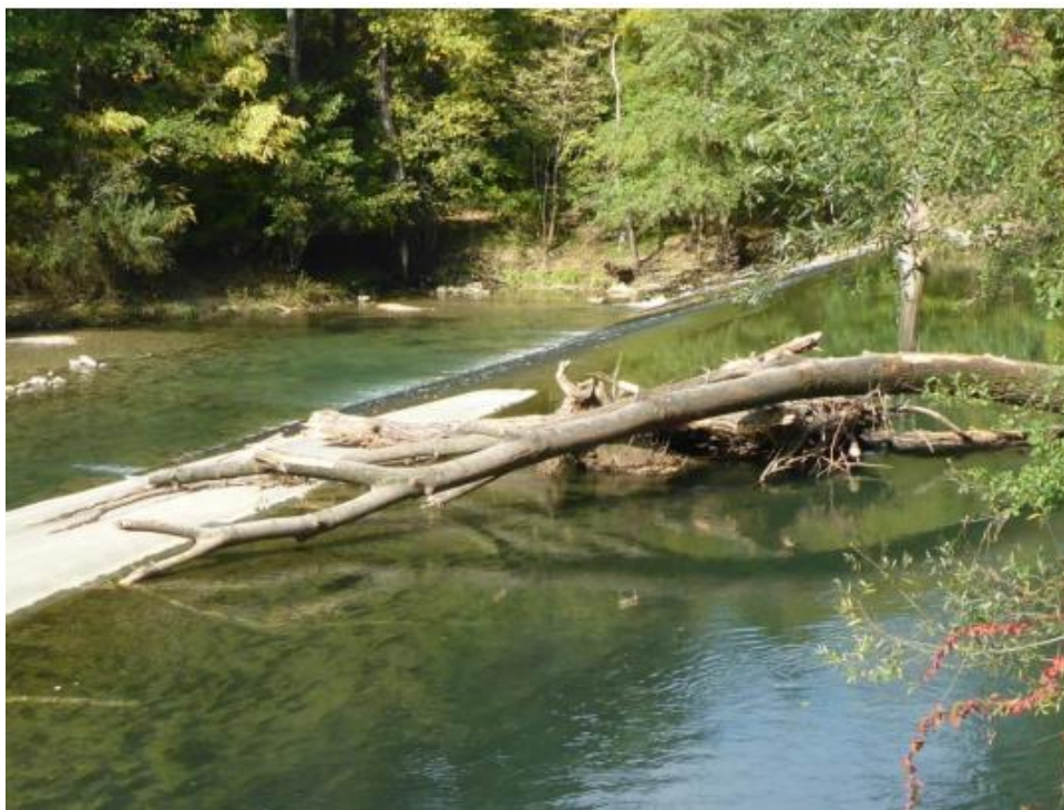
Image 6: Dam at Pikel.
