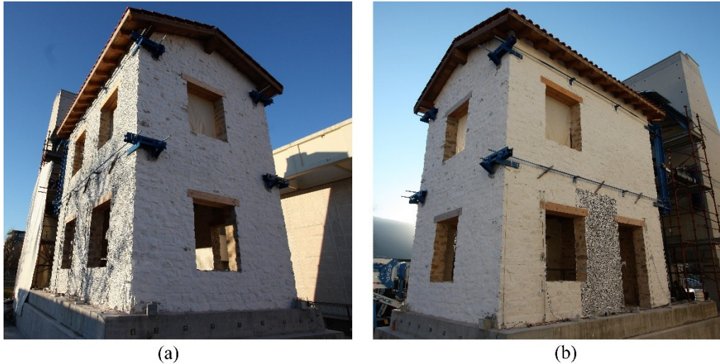
Fig. 1. View of the unreinforced test building: (a) East and North walls; (b) North and West walls.
