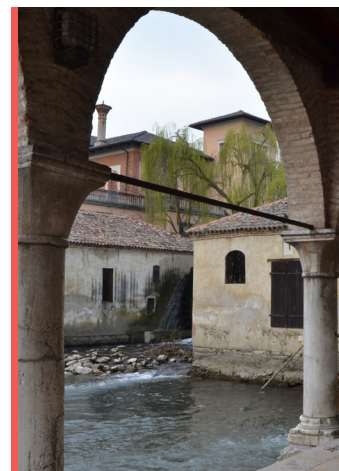
Portogruaro, two disused mills now housing an art gallery
