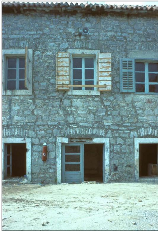
Fig. 17: Building sank 1m into liquefied soil.
