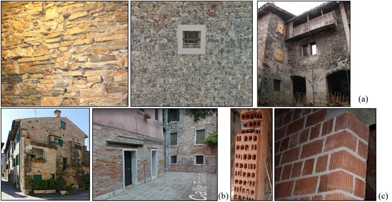
*Fig. 7: Masonry typologies in the Program area: stone (a), solid bricks (b) and hollow bricks (c).*
