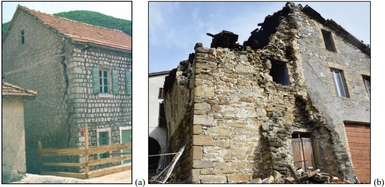
Fig. 9: Loss of structural integrity: a) separation of perimeter walls (Montenegro, 1979), b) insufficient connection to floor structures (Borgo, 2016).
