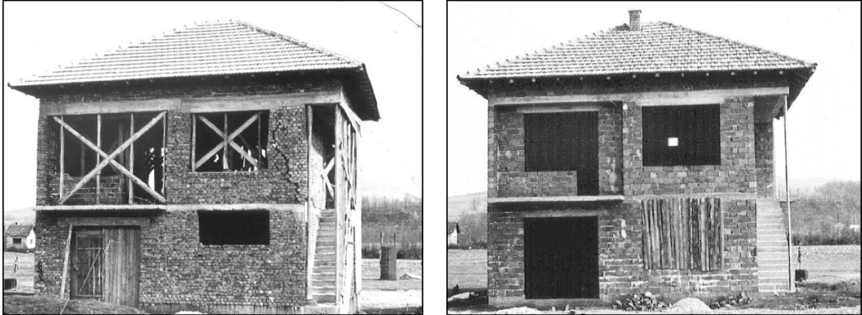
*Fig. 36: Two nearly identical structures after earthquake. Building from solid bricks and poor mortar on the left damaged, whereas building from hollow clay blocks and good mortar did not. Shot after Banja Luka 1969 earthquake. Photos courtesy of prof. Tomažević.*
