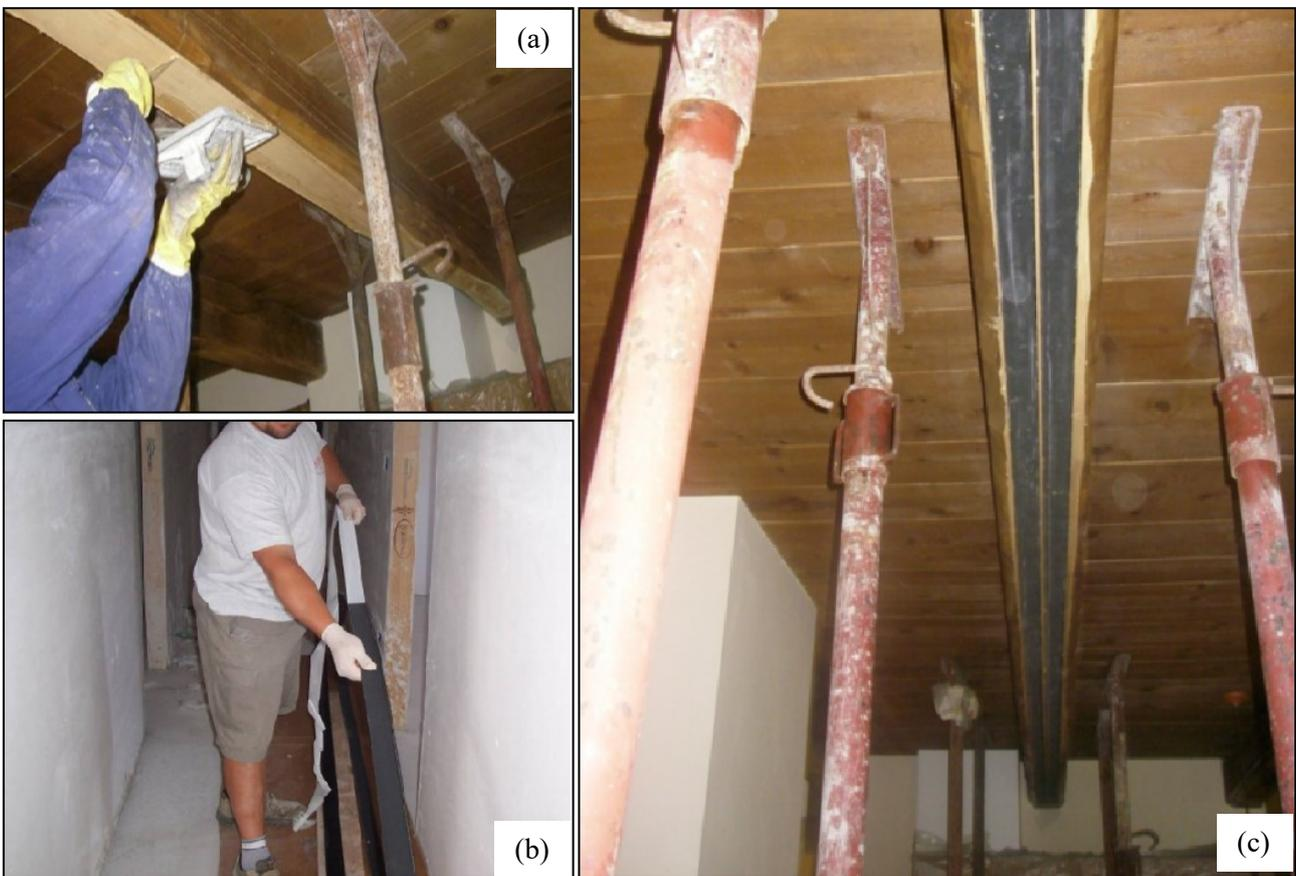
*Fig. 64: Wooden beam strengthening with the use of an FRP pultruded sheet: applying of a special thixotropic epoxy resin in the beam groove (a); peeling of the dust protection ply from the FRP plate (b), positioning of the pultruded sheet (c)*
