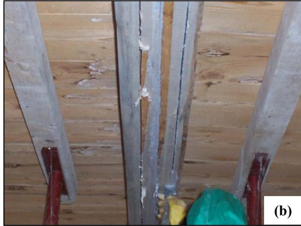
*Fig. 35: Propped ceiling joists strengthened by carbon fibre strips.*
