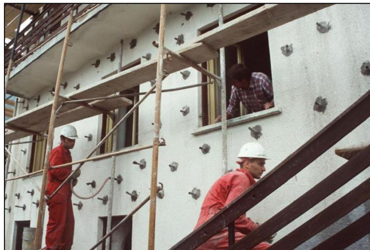
Fig. 39: Injecting stone masonry in practice<sup>5</sup>.
