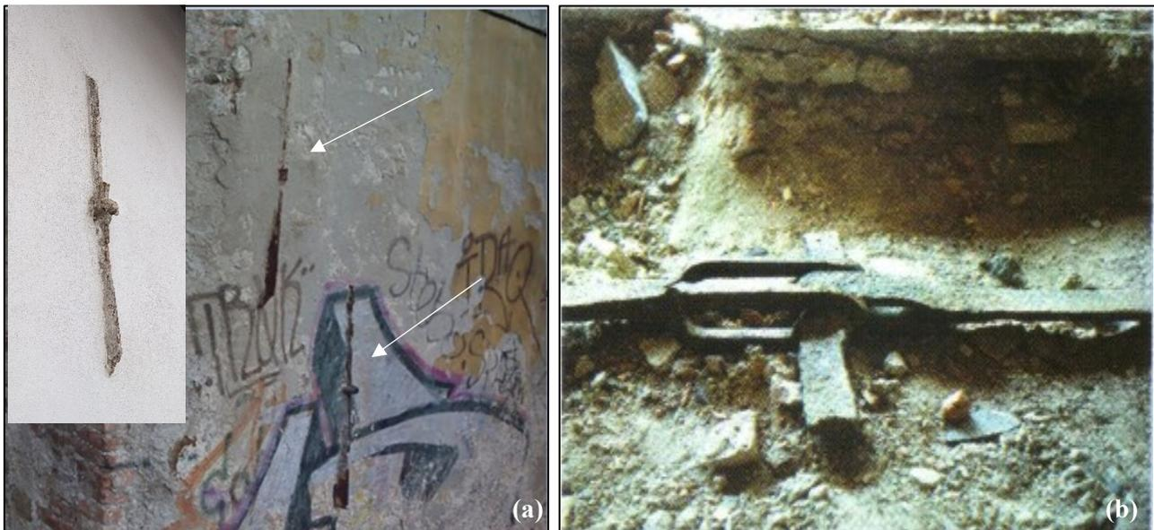
Fig. 19: Anchors of steel ties on the façade (a), iron tie from XVII century house in Ljubljana (from Tomažević, 2009) (b).
