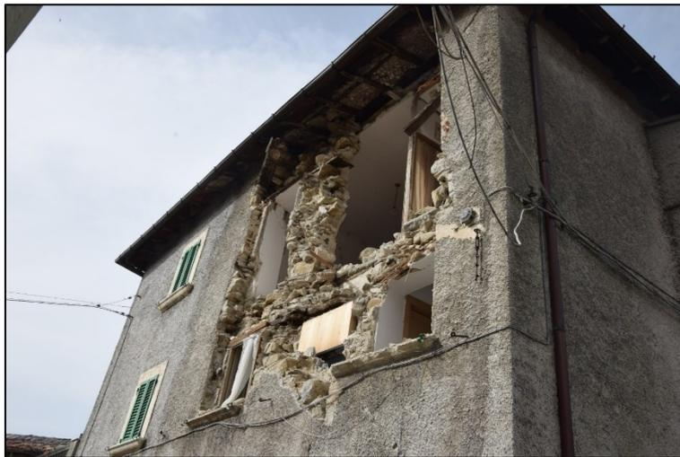
*Fig. 16. Out-of-plane failure of a two-wythe wall (Borgo, 2016).*
