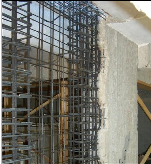
Fig. 20: Adding walls to an existing structure<sup>4</sup>.
