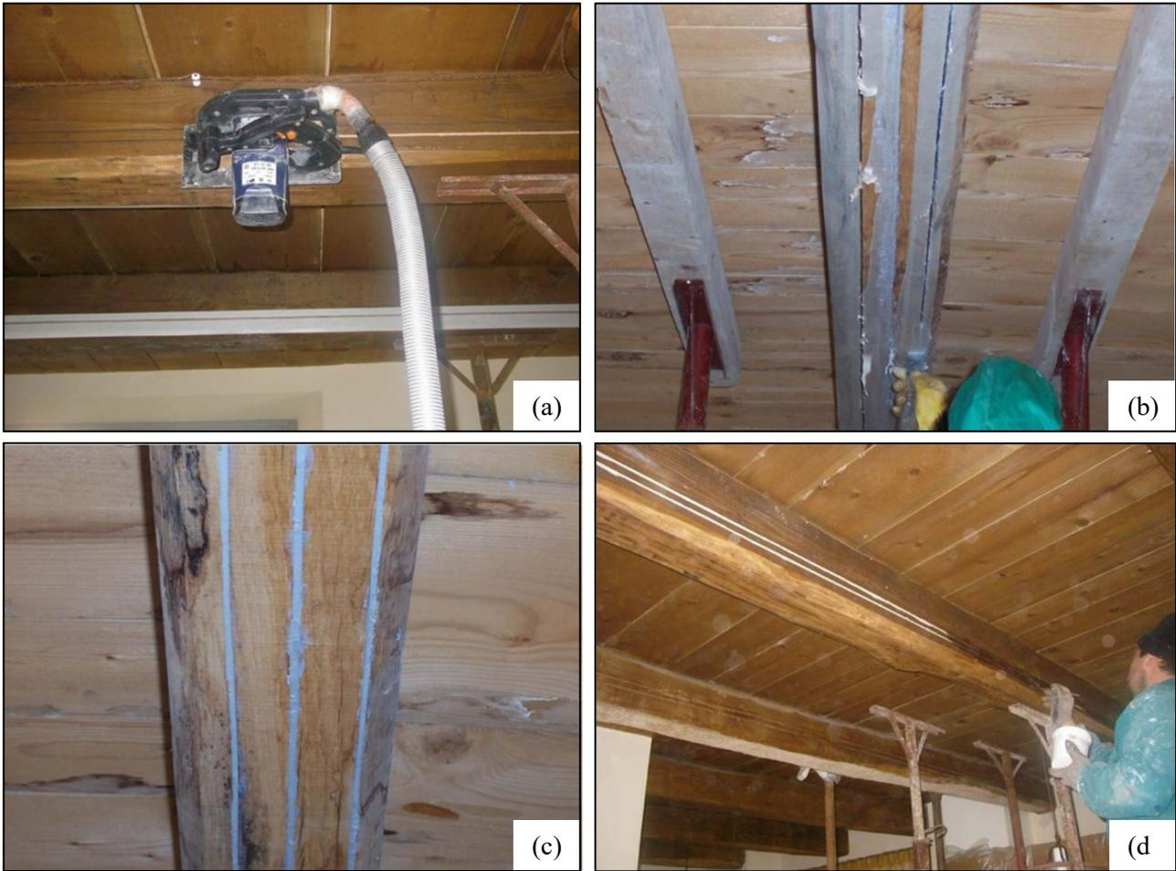
Fig. 65: Intervention through FRP sheets: carving the notches with a wood cutter (a), manual removal of the excess resin (b), positioning of the sheets (c and d)
