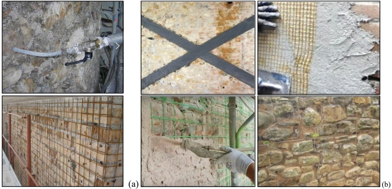
Fig. 37: Strengthening of existing masonry performances. Traditional grouting and RC coating (a). Modern techniques (b) Clockwise from top left: CFRP glued strips, Fibre Reinforced Cementitious Matrix (FRCM), repointing with steel strands and preformed GFRP mesh embedded in lime mortar.
