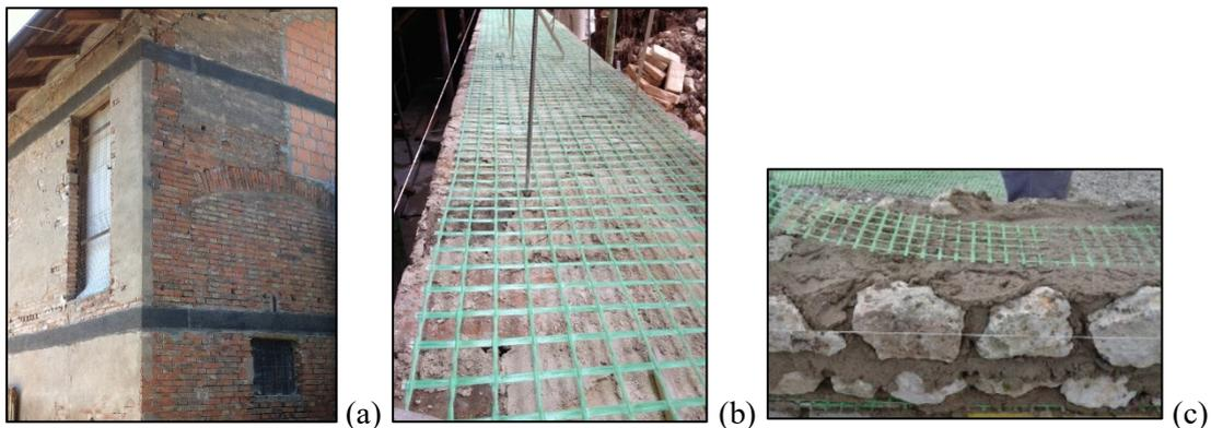
Fig. 26: CFRP ties at floor levels (a), GFRP top tie in a brick (b) and a stone masonry wall (c).
