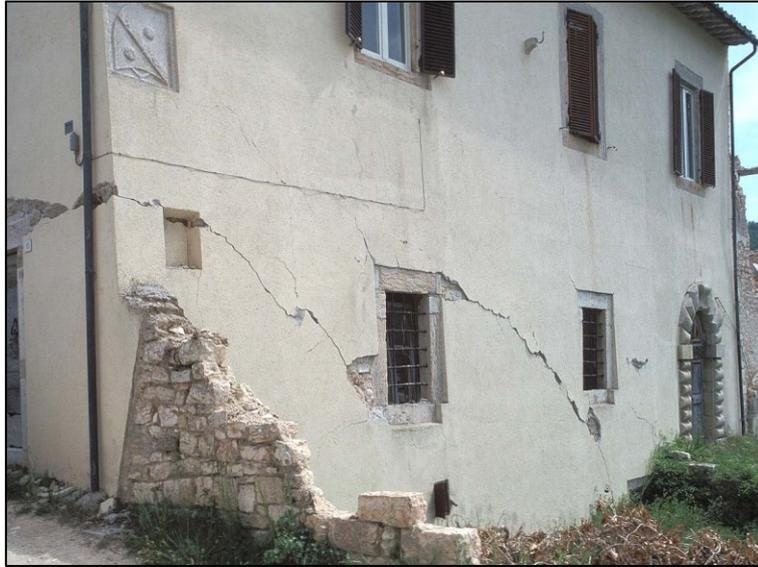
*Fig. 13: Diagonal shear damage (Umbria, 1997)*
