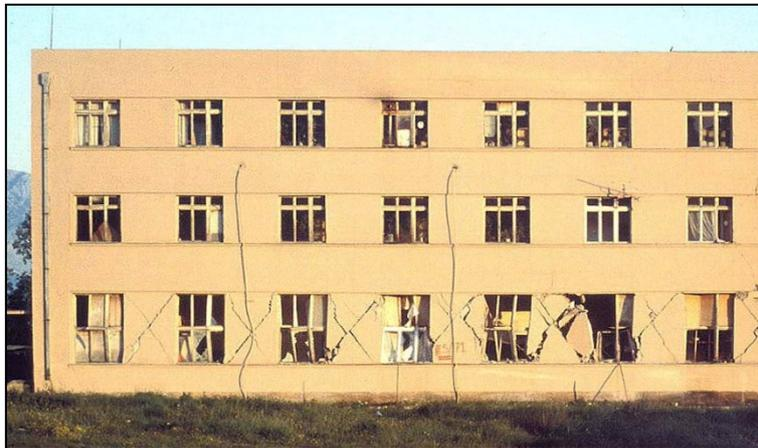
*Fig. 14: Typical diagonal shear damage in piers of ground storey (Budva, 1997)*
