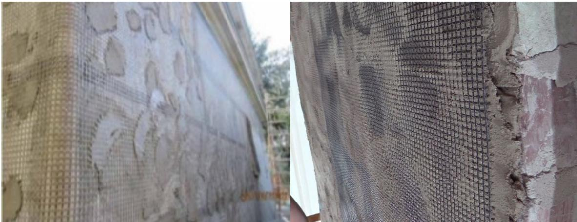
*Fig. 72: Strengthening technique: FRCM system*
