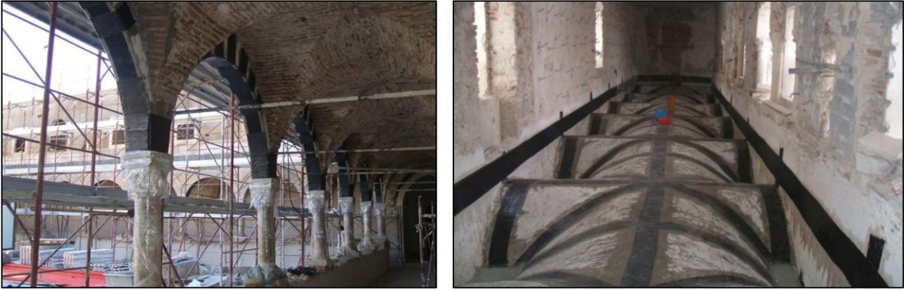
Fig. 43: Externally bonded FRP strips in arches (left) and vaults (right).
