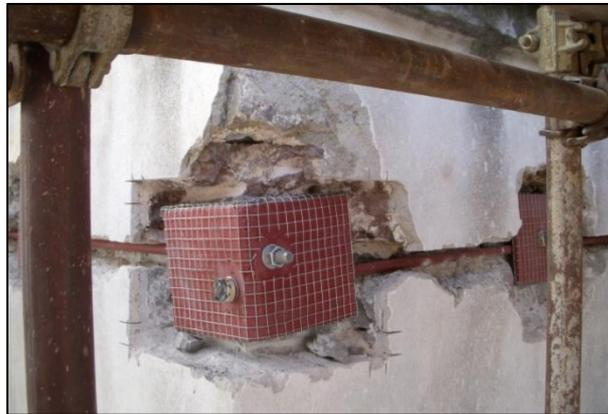
*Fig. 22: Ties and steel anchor plates at the corner.*
