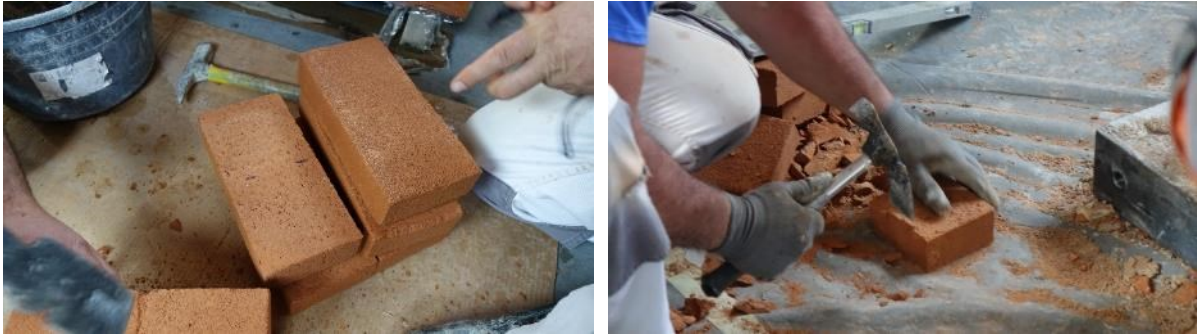
Fig. 2: Sorted bricks (left) and hammering in halves (right).
