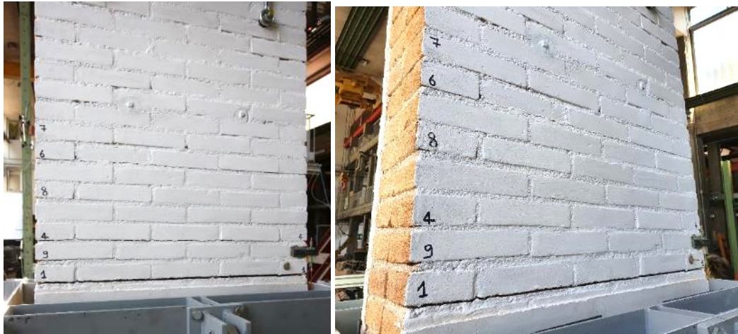
Fig. 92: Cracks on the unstrengthened side.
