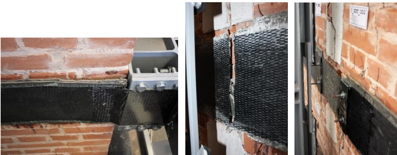
Fig. 164: crack configuration during the test – (a) unreinforced side middle section at step 6 (-4.0 mm); (b) upper part of the middle section on the reinforced side at step 7 (+5.0 mm); (c) vertical cracks outside of the middle section, on the left part at step 10 (+15.0 mm)
