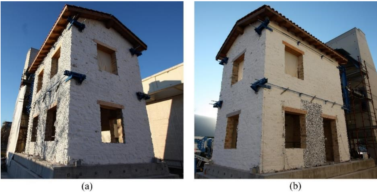
Fig. 173: View of the unreinforced test building: (a) East and North walls; (b) North and West walls
