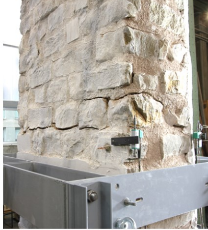
Fig. 80: Cracks on the unstrengthened side at u = -22.0 mm
