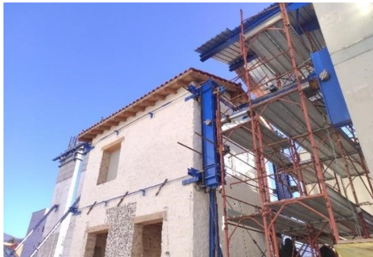
Fig. 179: System for the application of horizontal load.
