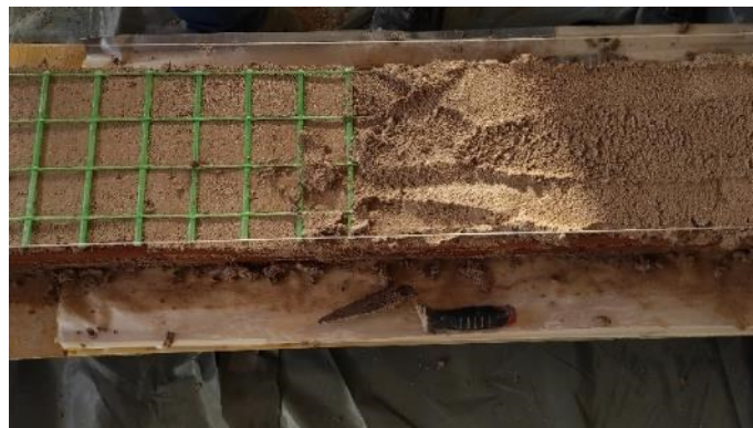
Fig. 147: Mesh embedded in the bed joint.
