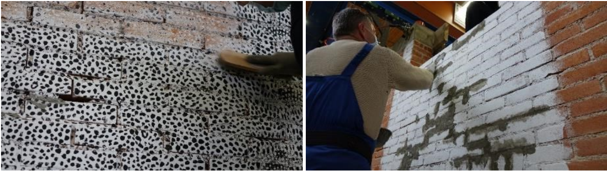
Fig. 19: Cleaning the surface (left) and sealing the cracks (right).
