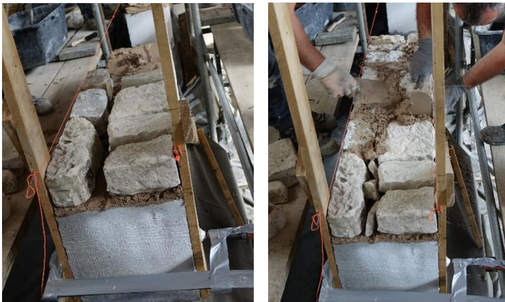
Fig. 13: Construction of stone masonry wall.
