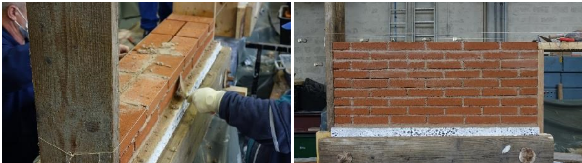
Fig. 15: Filling joints (left) and specimen during construction (right).
