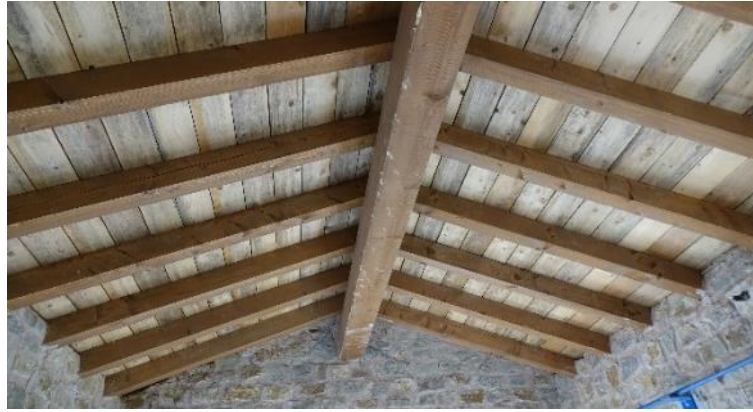
Fig. 175: Roof of the pilot building
