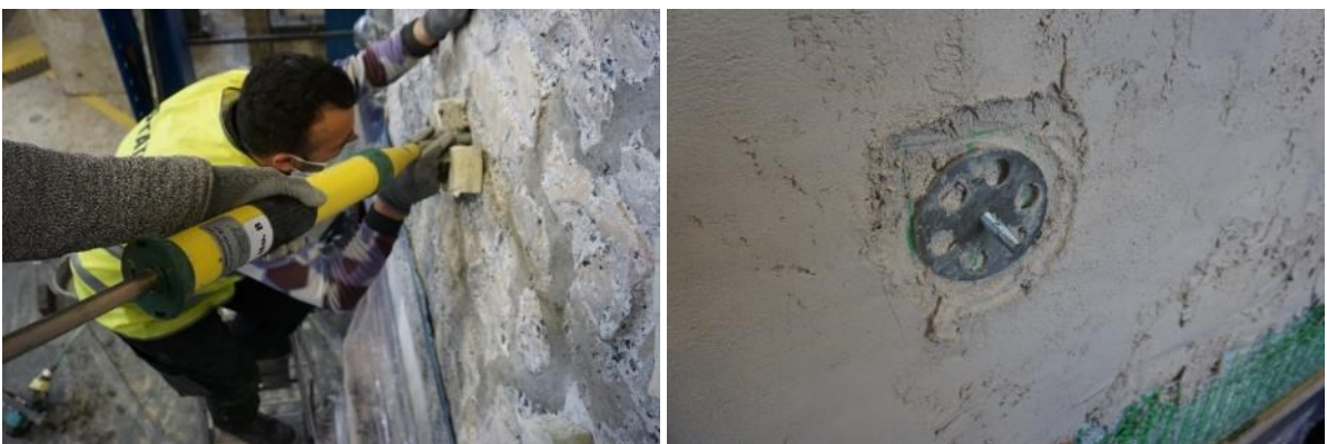
Fig. 18: Injecting TX100 grout (left); installed anchor plate (right).
