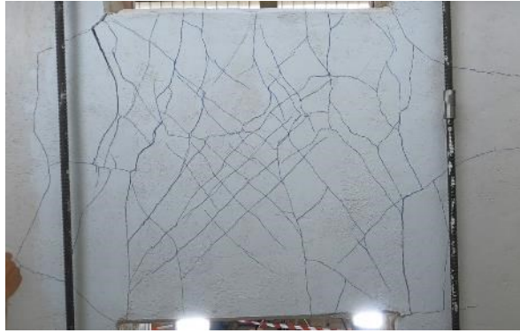
Fig. 114: Crack pattern at maximum resistance
