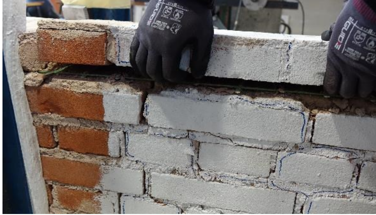
Fig. 149: Top row separated from the wall at collapse.
