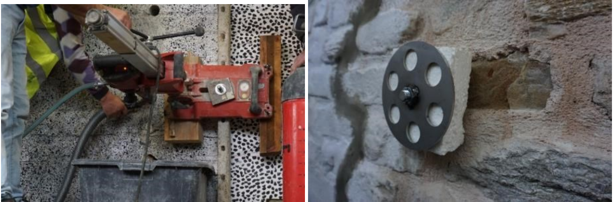
Fig. 17: Drilling of 50 mm holes (left); temporary fixing of diaton (right)
