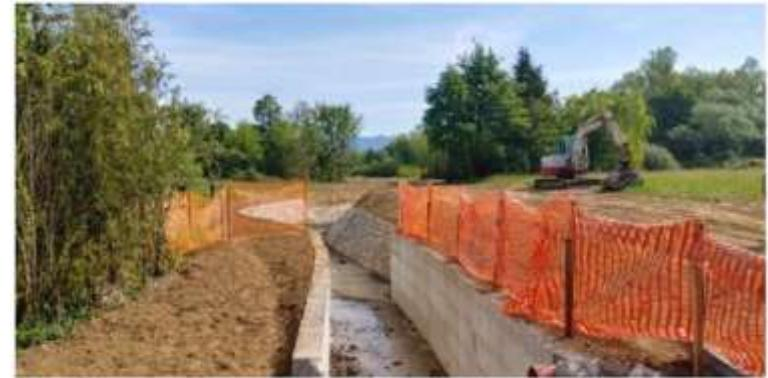
Fig. 10 U-shaped concrete channel construction
