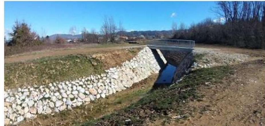
Fig. 11 Adjustment of the culvert into a reinforced concrete bridge
