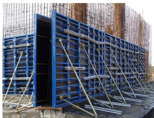
Figura 4: Cassaforma in metallo compensato ([www.ceta.it](http://www.ceta.it))
